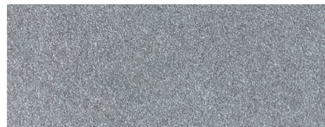
“Metallic Plaster”, 1st coat SWS 404 with plastic trowel; second coat SWS 404 and Swahili silver with plastic trowel.
